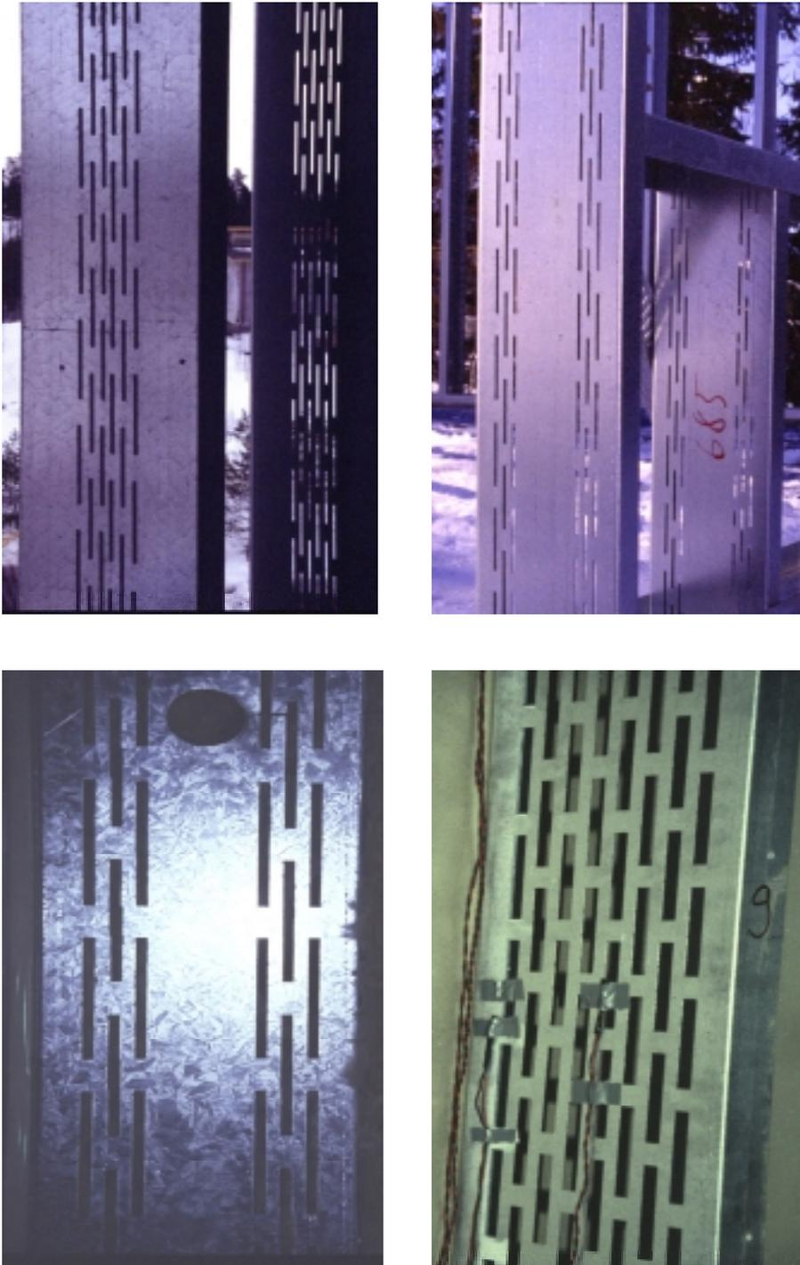
*Figure 2. Thermoprofile alternatives. Profiles in the top row were used in Villa 2000 built for the Tuusula housing fair 2000 (left), and in Ylöjärvi steel houses built for the Ylöjärvi housing fair 1996 (right). Other two examples were manufactured for testing purposes.*
