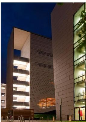
The architectural concept for the redesign of the building envelope was characterised by its former use. Horizontal aluminium sheets were used for the façade, which vary in height and have a distance of 3 cm between each other. The entire curtain wall façade has a distance of approx. 60 cm to the load-bearing outer skin of the building made of aerated concrete elements. The orange light behind the curtain wall is intended to symbolize the glow of the coal.
